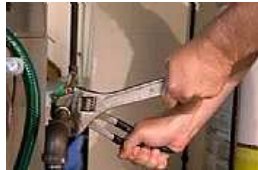
Prevent Basement Condensation
